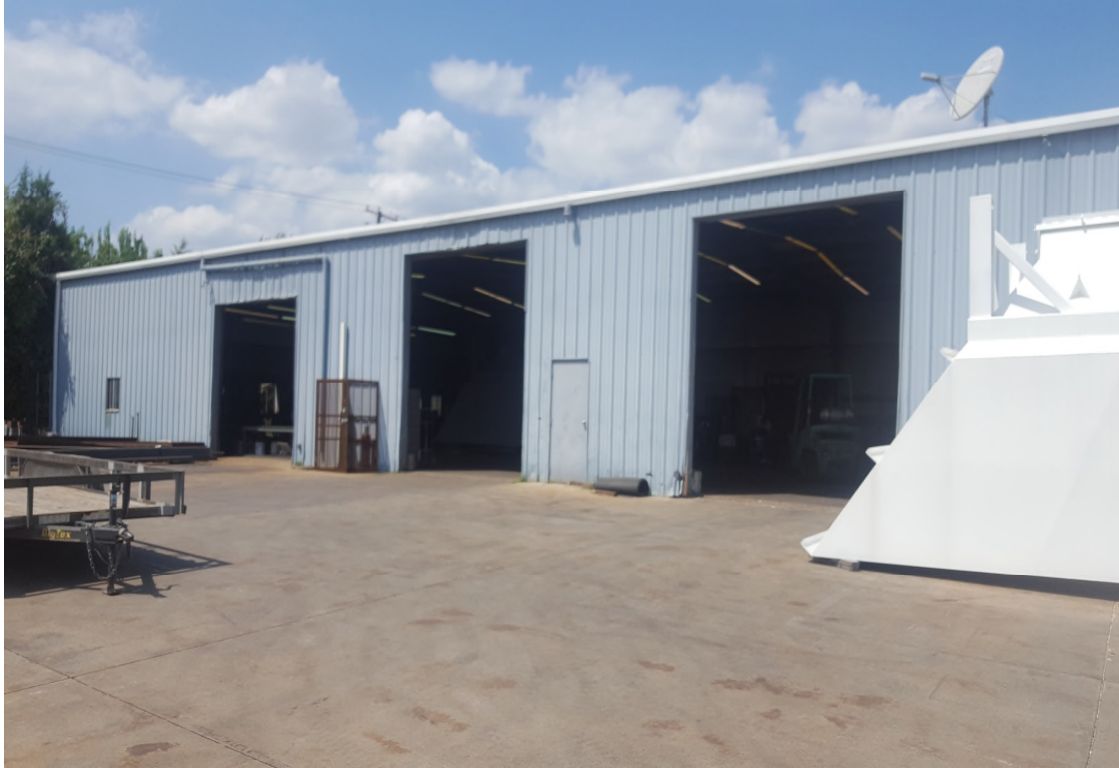
Side View/Parking Area
